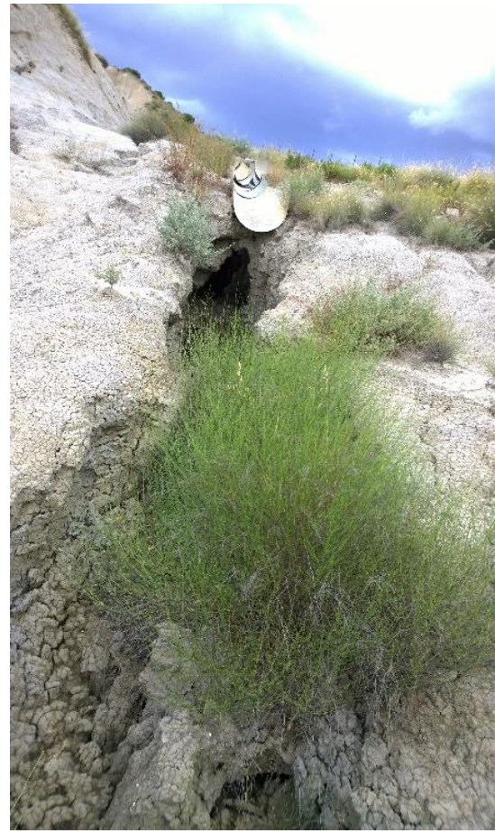
Fig. 3 – Drain in dump at Tursi (Italy)
